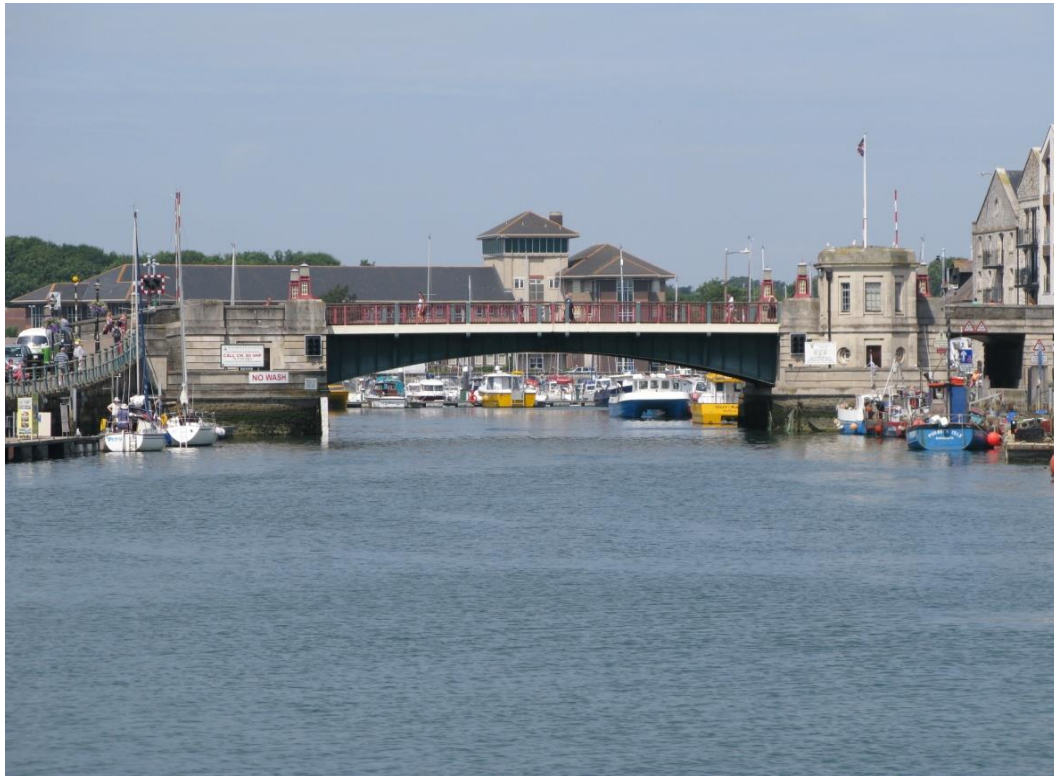
Figure 3. Town Bridge closed
