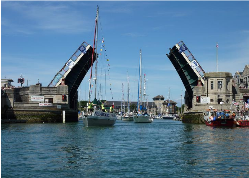
Figure 4. Town Bridge fully opened
